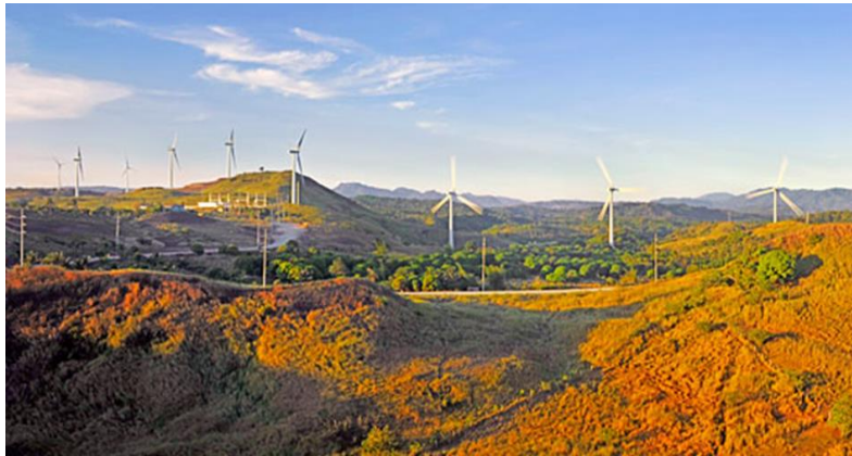
67.5 MW Wind power project located in Pililia, Rizal
