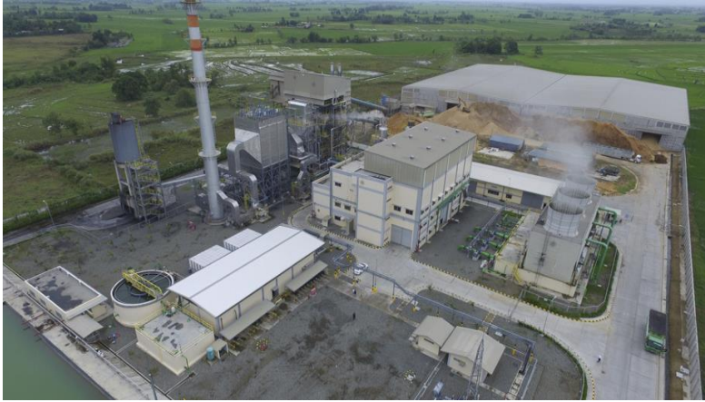
20 MW Biomass Rice husk-fired project located in Alicia, Isabela
