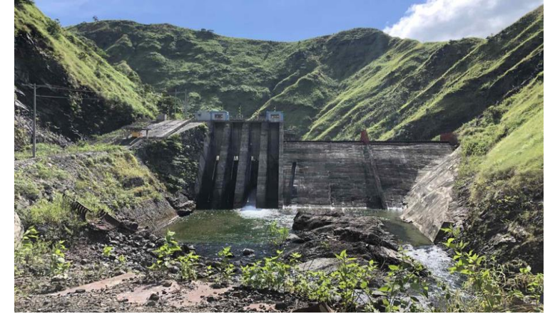
8 MW Mini Hydro Power plant located in Bugasong, Antique
