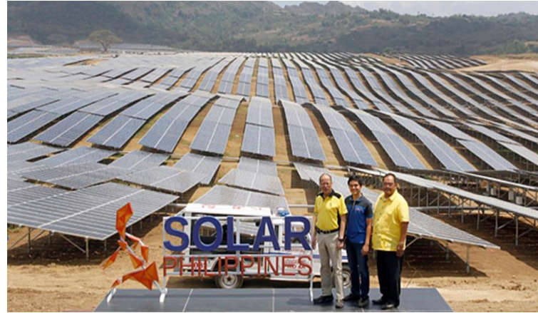
63.29 MW Solar Power Farm located in Calatagan, Batangas
