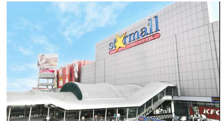
Retrofitting made to HVAC & Lighting system for Starmall, Alabang in 2013. Awarded by UNFCC for the EE Category for SEF Awards in 2014.
