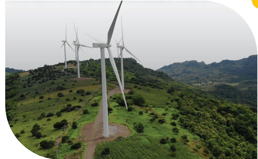
75 MW Sidenreng Rappang (Sidrap) Wind Farm, South Sulawesi Photo by MEMR
