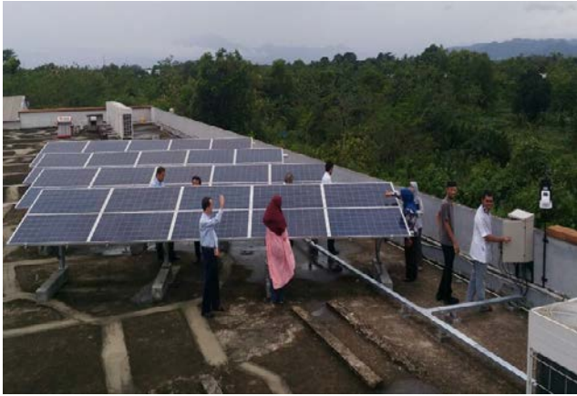
Smart microgrid 10 kWp PV rooftop Serpong
