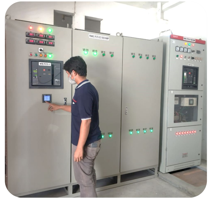
Ruang Panel MDP Solar Panel
