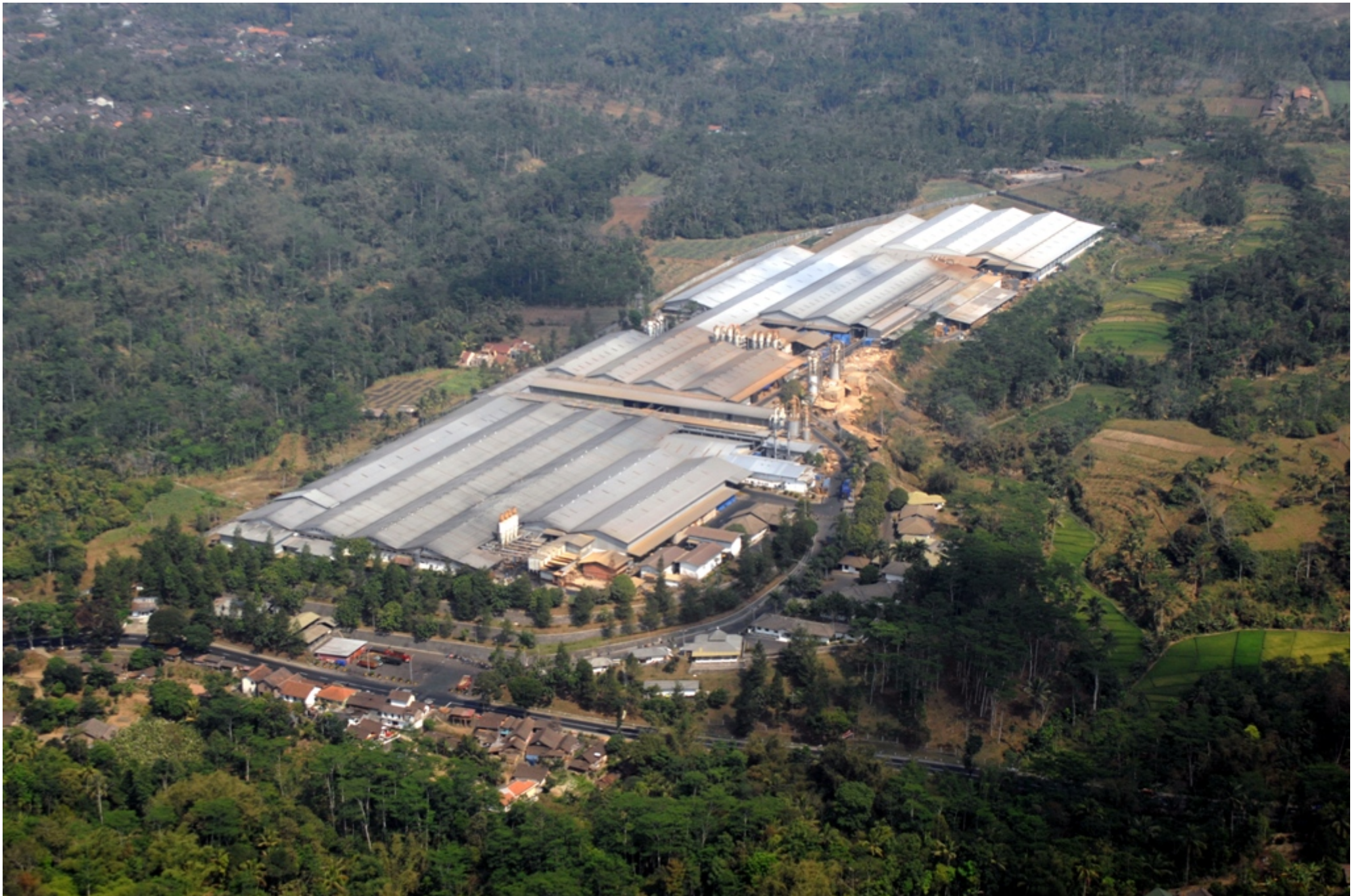
2 MWp of Rooftop Solar Photovoltaics Construction by ATW Solar Indonesia in PT. Tanjung Kreasi Parquet Industri, Temanggung
