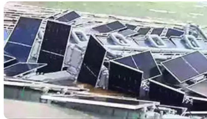
The floating solar plant at Omkareshwar Dam after a storm
